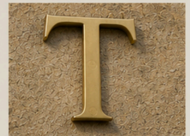
Detail of finish and fixing
